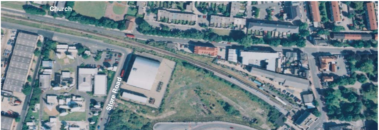
North Woolwich Portal
